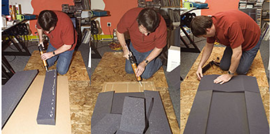
Following a quick trip to B&Q, Paul constructed an acoustic panel using a sheet of MDF, some adhesive, and elements of a Primacoustic foam room-treatment kit.
