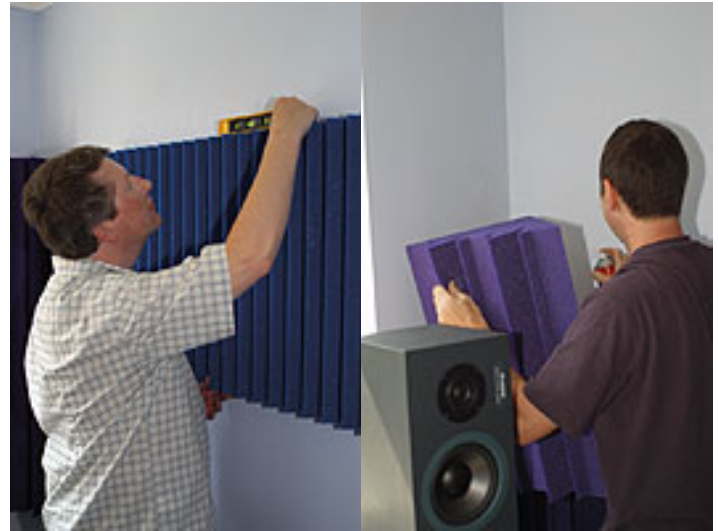
Hugh installs the newly made wall panels, using a spirit level for a neat result, while Paul carefully sticks acoustic foam bass traps directly into the front corners of the room using more spray adhesive.
