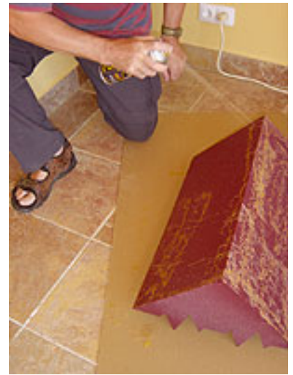
The first step towards reducing the excess reverberation in Dave's room was to install several Auralex acoustic foam panels and corner traps using contact adhesive spray.
