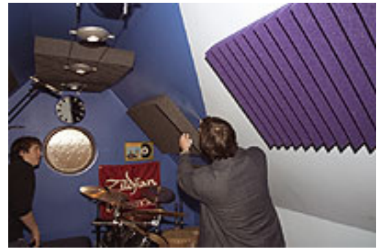
As an attempt to dry up the sound further, Paul fixed more foam to the wall behind the drums.
