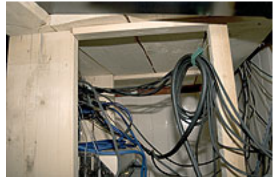
Once the mains cables had been re-organised, the audio wiring was tied up out of the way of them using cup hooks and Velcro cable ties.
