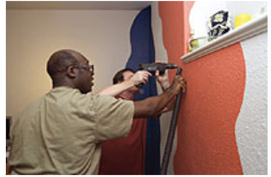
Aniff held a vacuum cleaner to catch the dust while Paul drilled holes for mounting the acoustic-foam panel he'd just put together. Once the hole was drilled, it was fitted with a wall plug to accept the mounting screw. A picture bracket was then screwed to the back of the panel so that it could be fitted to the wall screw's head.
