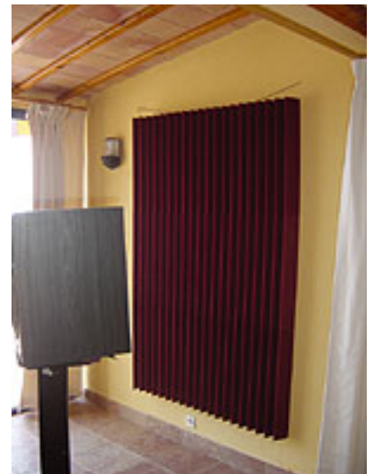
A large area of foam treatment was created by sticking multiple foam panels to MDF, and this
