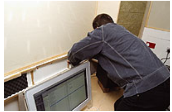
A few offcuts of acoustic foam were pressed into service to reduce reflections from the wall behind the monitors.
