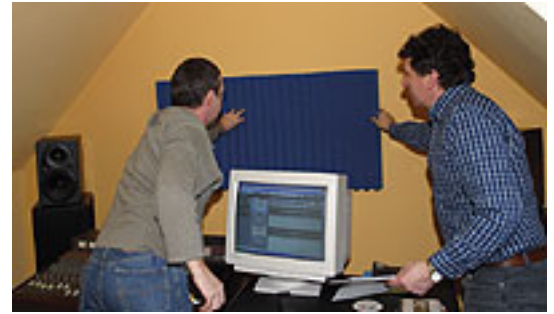
Temporarily placing a panel of acoustic foam behind the monitors facing the monitoring position confirmed that this would improve the sound by avoiding strong reflections from the wall.
