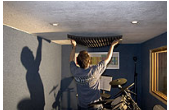
The final remaining foam panel was placed on the ceiling in the live room, above where Brett was planning to set up his mic for vocal recording.
